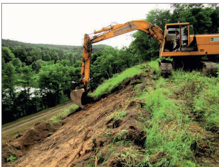
Photograph 71. Removal of the top layer of soil in the Trutwiniec sub-area (Dolna Odra site) (by K. Barańska)
