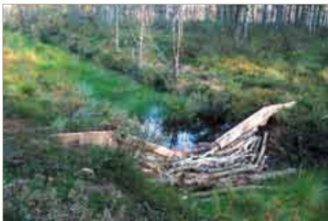
Fot. 8. W ramach projektu wybudowano kilkaset zastawek. Some hundreds damming barriers have been built in frames of project.
